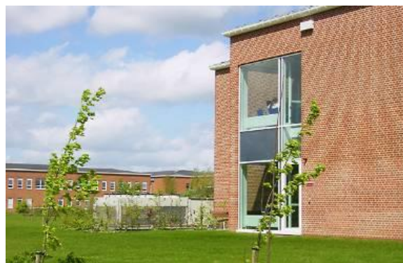
Photo. 5: A 60 kW Hydro-Carbon chiller serving a hospital in Aarhus. Installed 2003. [Today, there are chairs and tables arranged nearby for smokers.]
