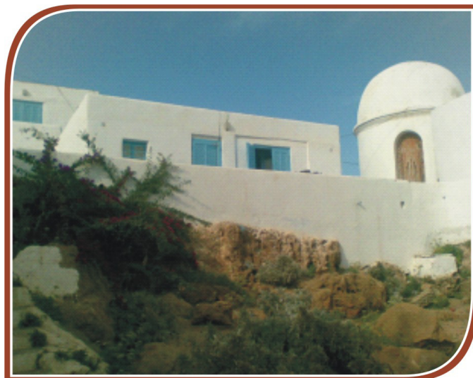
Traditional architecture is an important criteria for ecolabelling
